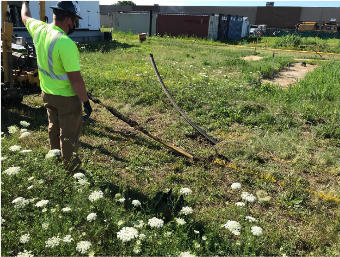
Figure 11: Field test HDD installation in progress
